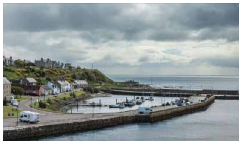
Surveys carried out at low tide along with manual depth measurements from a local boat have shown that the harbour is clogged up with mud and large banks of stones have built up on the channel leading out to sea.
