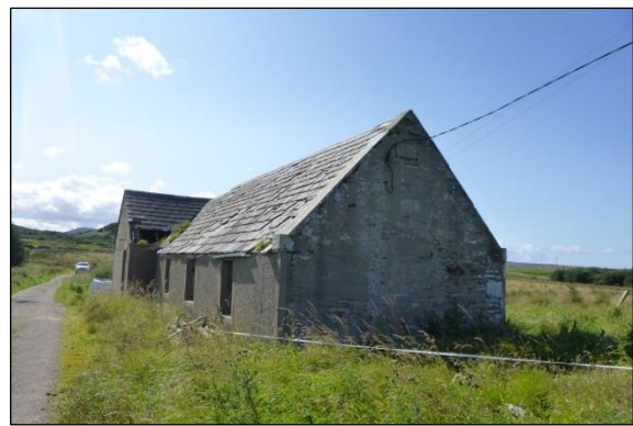
Photo 4 Moderate to High Potential Bat Building (Milton)
