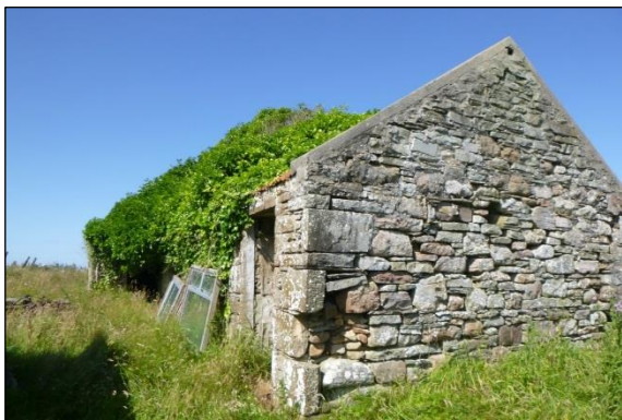
Photo 5 Moderate to High Potential Bat Building (Milton)
