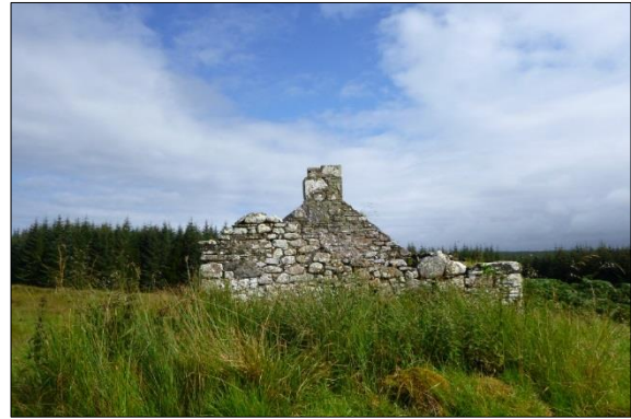
Photo 2 Building with hibernation potential
